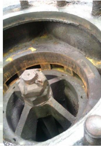
Figure 1 Intermediate Pressure valve assembly
